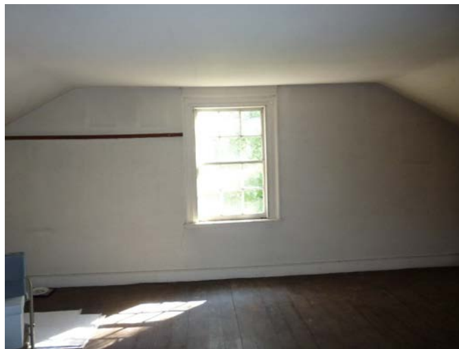
Figure 29. South room in attic, looking south (2016).
