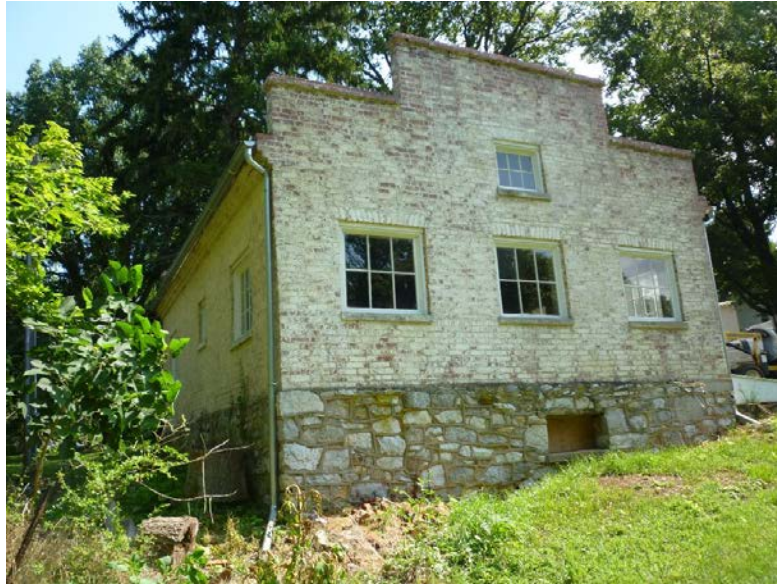
Figure 33. Southwest view of garage (2016).
