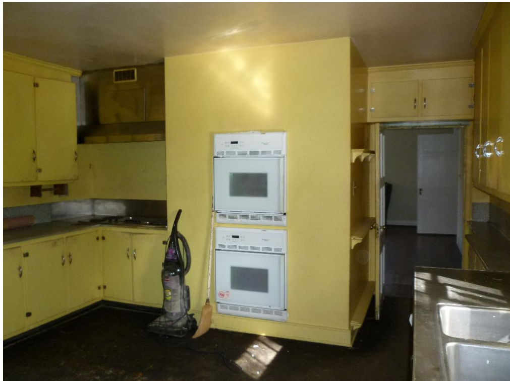
Figure 16. The former kitchen (Room 106) before demolition of the finishes. View looking north into Room 105 (2016).
