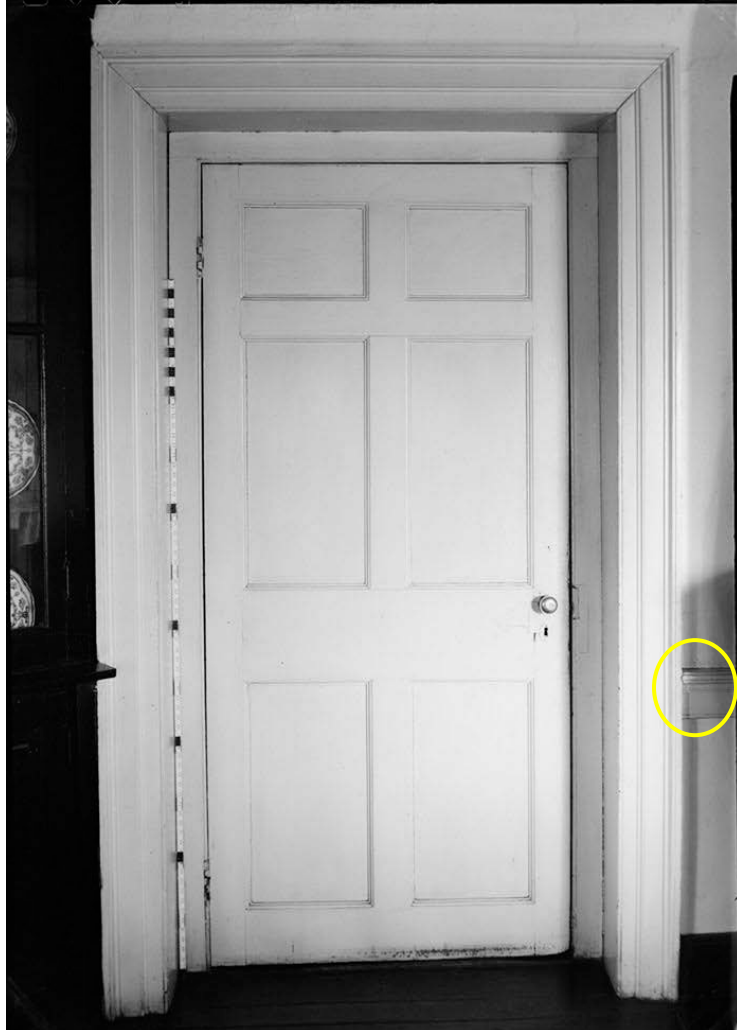
Figure 6. Room 105, Period I exterior door and door casing, showing chair rail connecting to back band (HABS 1937 www.loc.gov/pictures/item/wv0090.photos.172243p/resource/ ).
