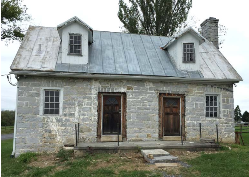
Figure 12. Two-room store at Belle Grove, Frederick County, Virginia; former bulkhead entrance to full basement located between the doorway and window on the right; dormers were a later addition (2016).
