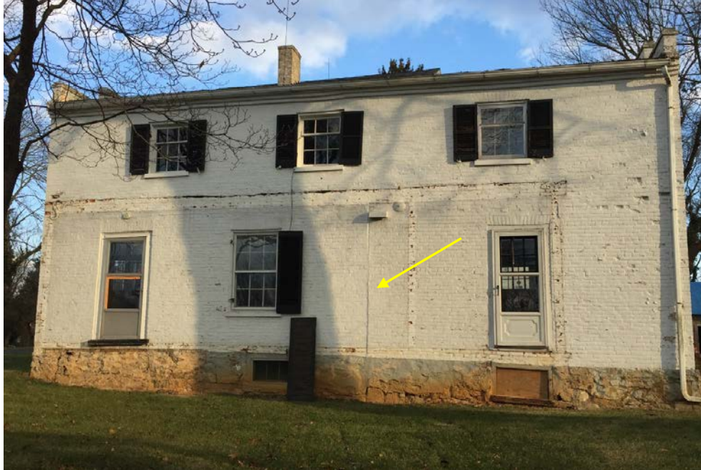
Figure 3. West wing, west elevation after removal of 20 th -century porch (2016): Period I one-story section on the left (north); Period II on the right; second floor added in Period III. The window and doorway in Period I section added; doorway in Period II section converted from an original window.
