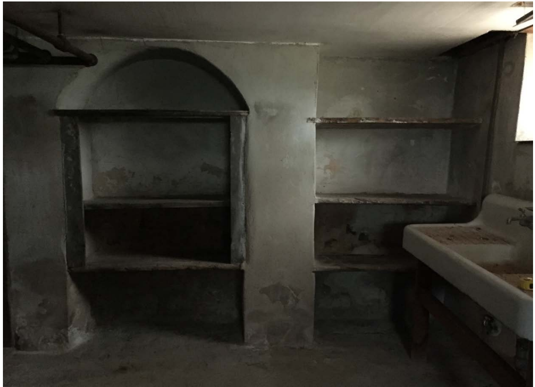
Figure 15. Built-in shelves within the relieving arch for the fireplace and in the niche between the arch and the southwest corner of the Period I basement (2016).
