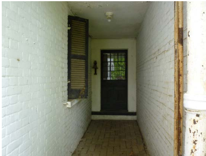
Figure 8. View of rear of west hyphen (2016).
