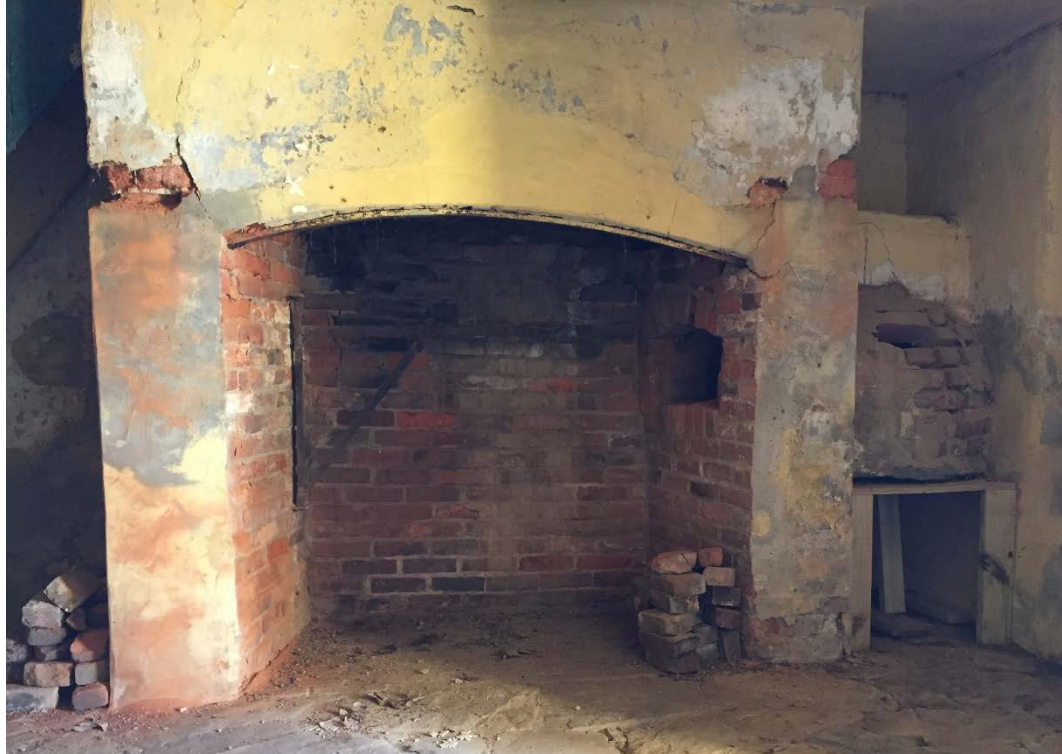
Figure 20. Fireplace and brick bake oven in kitchen (2016).
