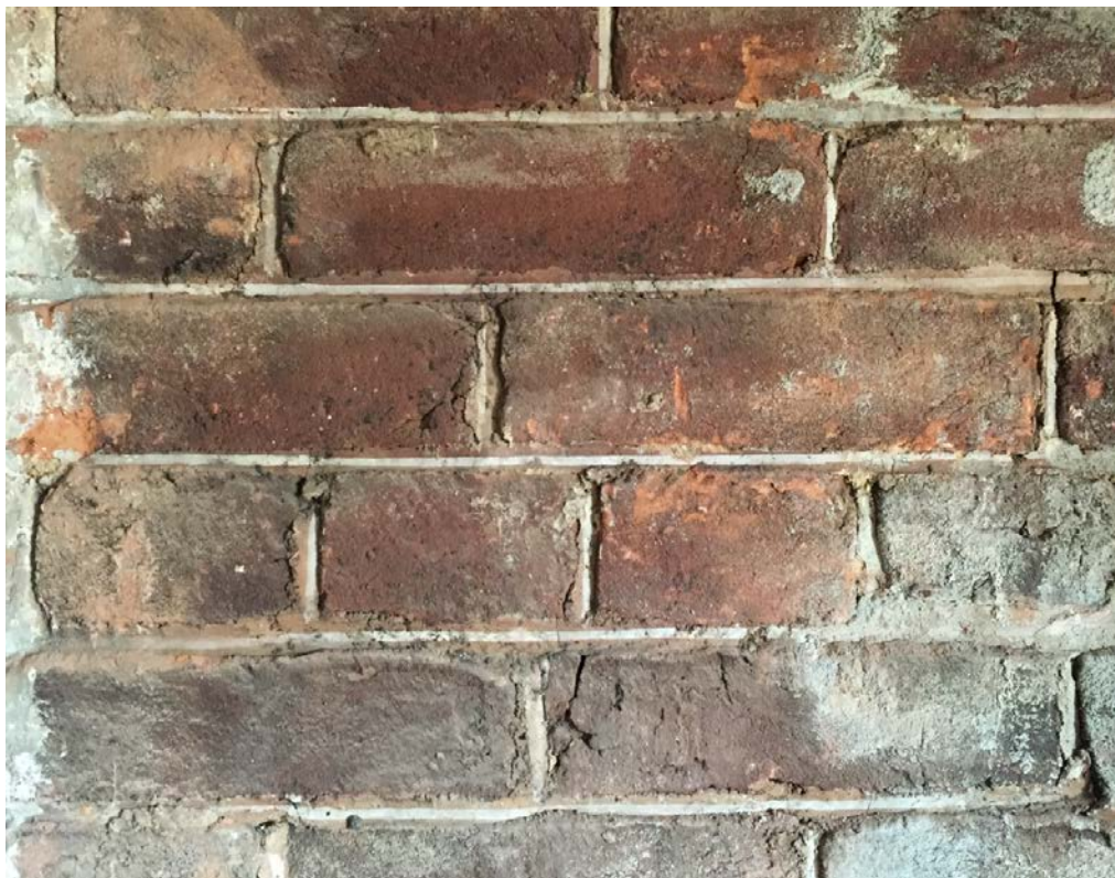
Figure 4. Ruled and penciled brick joints revealed on exterior face of Period I south wall, encapsulated within Period II Room 106 (2016).
