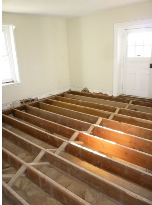
Figure 20. Room 109, with flooring removed (2016).
