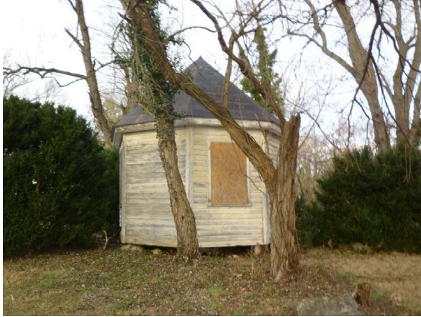
Figure 31. Southeast view of schoolhouse (2016).
