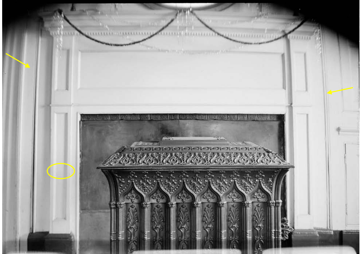
Figure 7. Fireplace and mantel in Room 105; vertical seams flanking mantel piece suggesting that the mantel was moved from another location; horizontal seam visible in the field of the panel on the lower left (HABS 1937, www.loc.gov/pictures/item/wv0090.photos.172244p/resource/ ).
