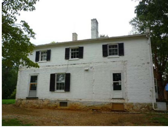
Figure 6. West view of west wing (2016), after the patio had been removed.
