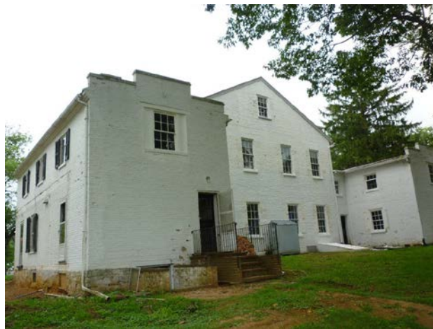
Figure 7. Southwest view of west wing (2016).
