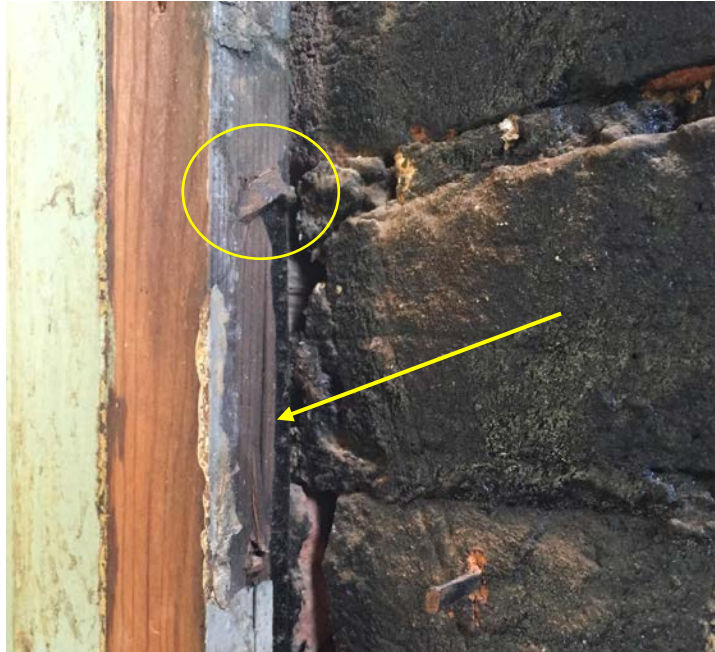
Figure 13. Paint ghost indicating square profile of chair rail found in Room 106; wrought L-head nail used to attach the chair rail, bent over and embedded in the side of the architrave (2016).
