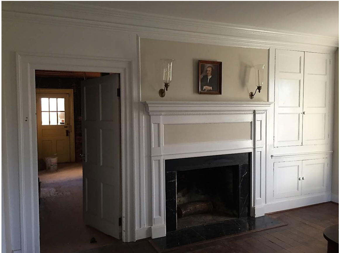
Figure 5. Room 105, south wall: doorway inserted in Period II; mantel piece a replacement; cabinet original to Period I (2016).
