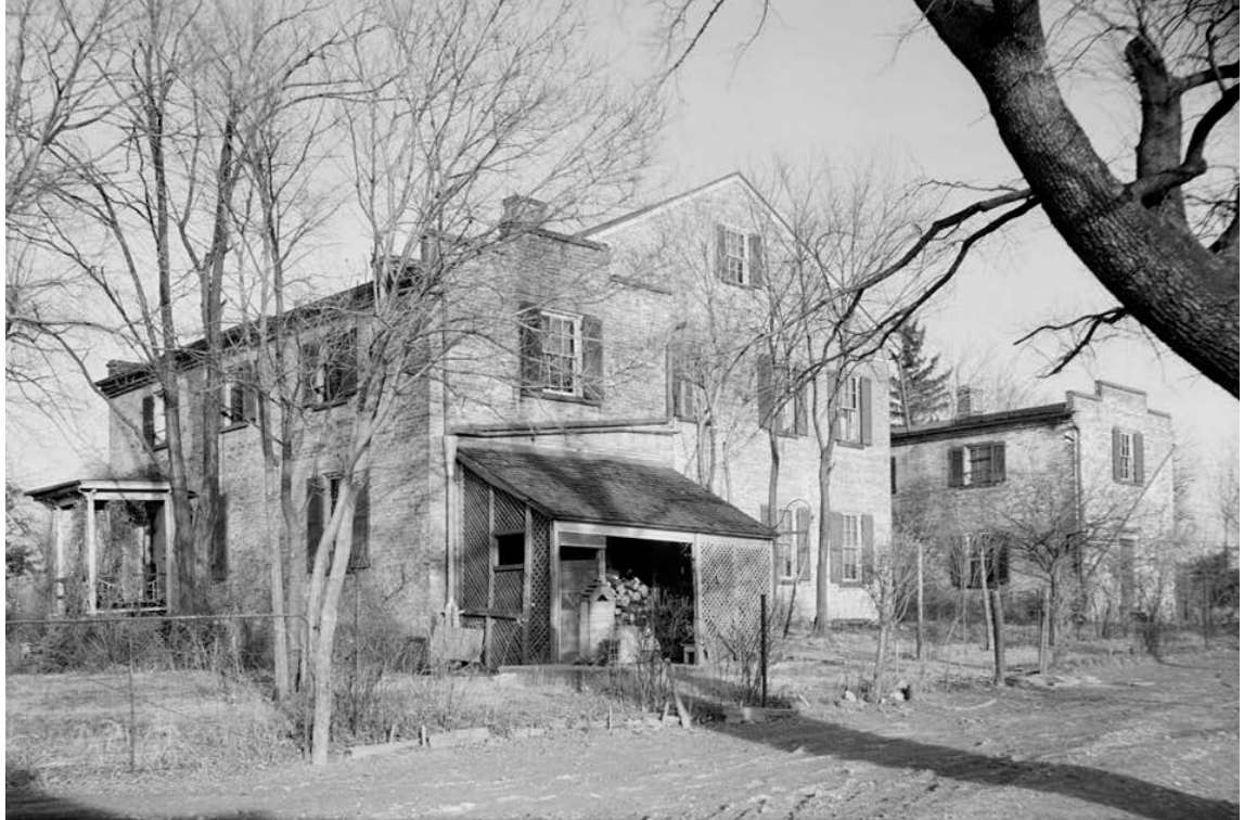
Figure 1. Happy Retreat from the southwest, west wing in the foreground; second floor, stepped gable parapets, porch and wood shed all circa 1842 and later (HABS 1937, www.loc.gov/pictures/item/wv0090.photos.172242p/resource/ ).
