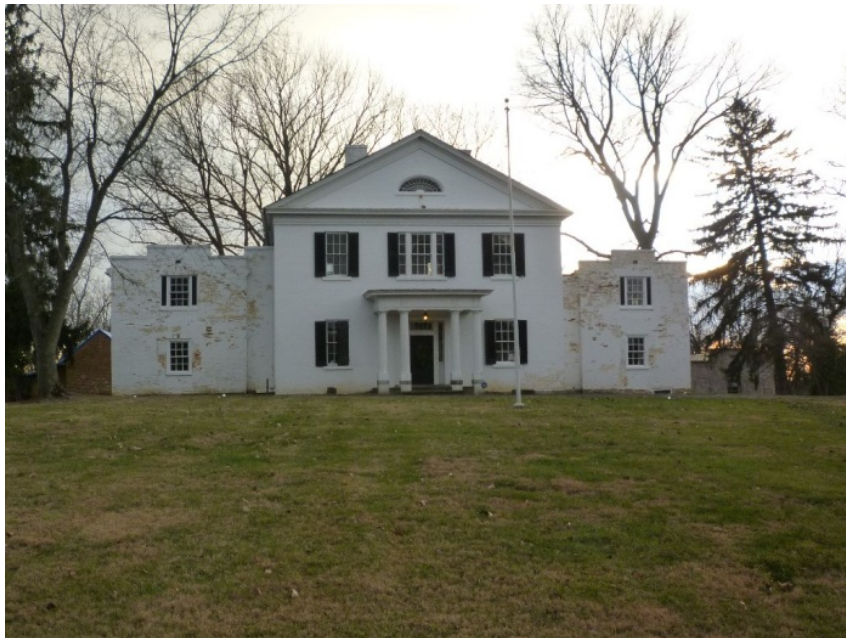
Figure 1. North view of house (2016).
