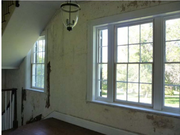
Figure 22. Stair at second-story landing (2016).
