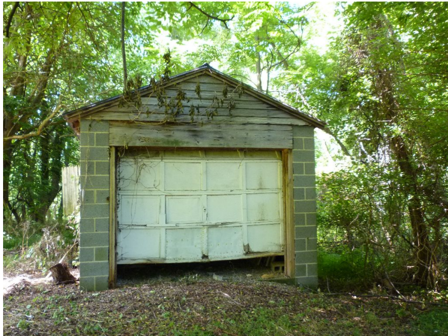
Figure 34. North view of former stable (2016).
