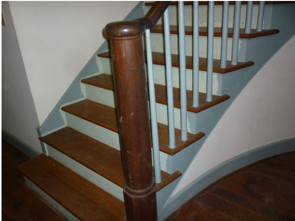
Figure 19. Staircase in east wing (2016).
