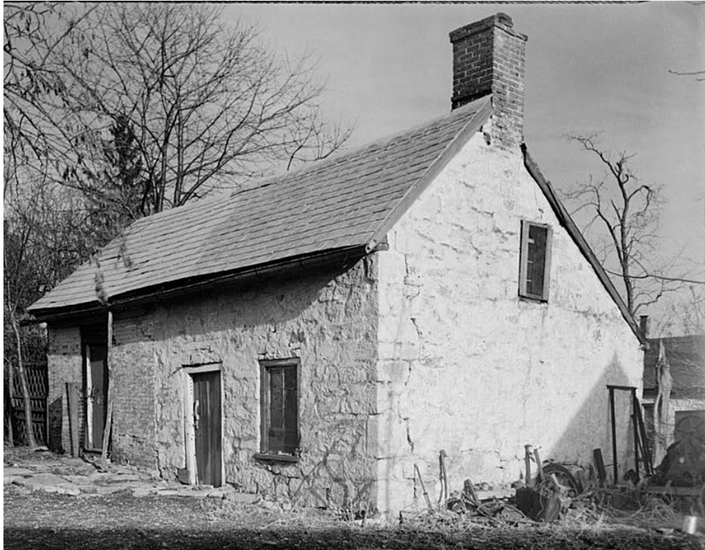
Figure 19. View of the brick smokehouse (left) and the stone kitchen; the second stone structure, with the centered chimney stack, is visible in the background (HABS 1937, http://www.loc.gov/pictures/item/wv0090.photos.172246p/resource/ ).
